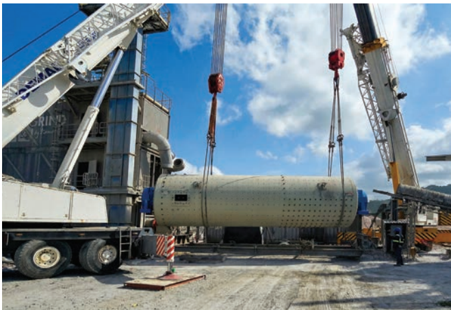
—Installation of the Plug&Grind® XL at the plant with the custom split bearing support system fully integrated.
