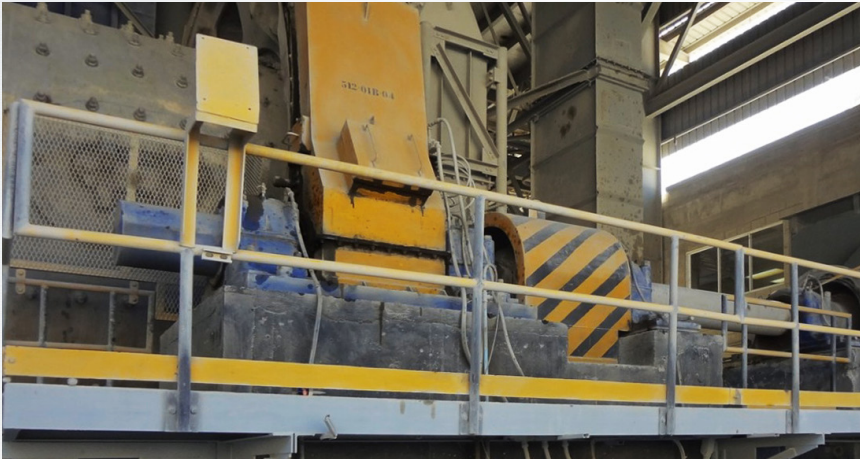
Picture of original Cementos Santo Domingo ball mill drive.
